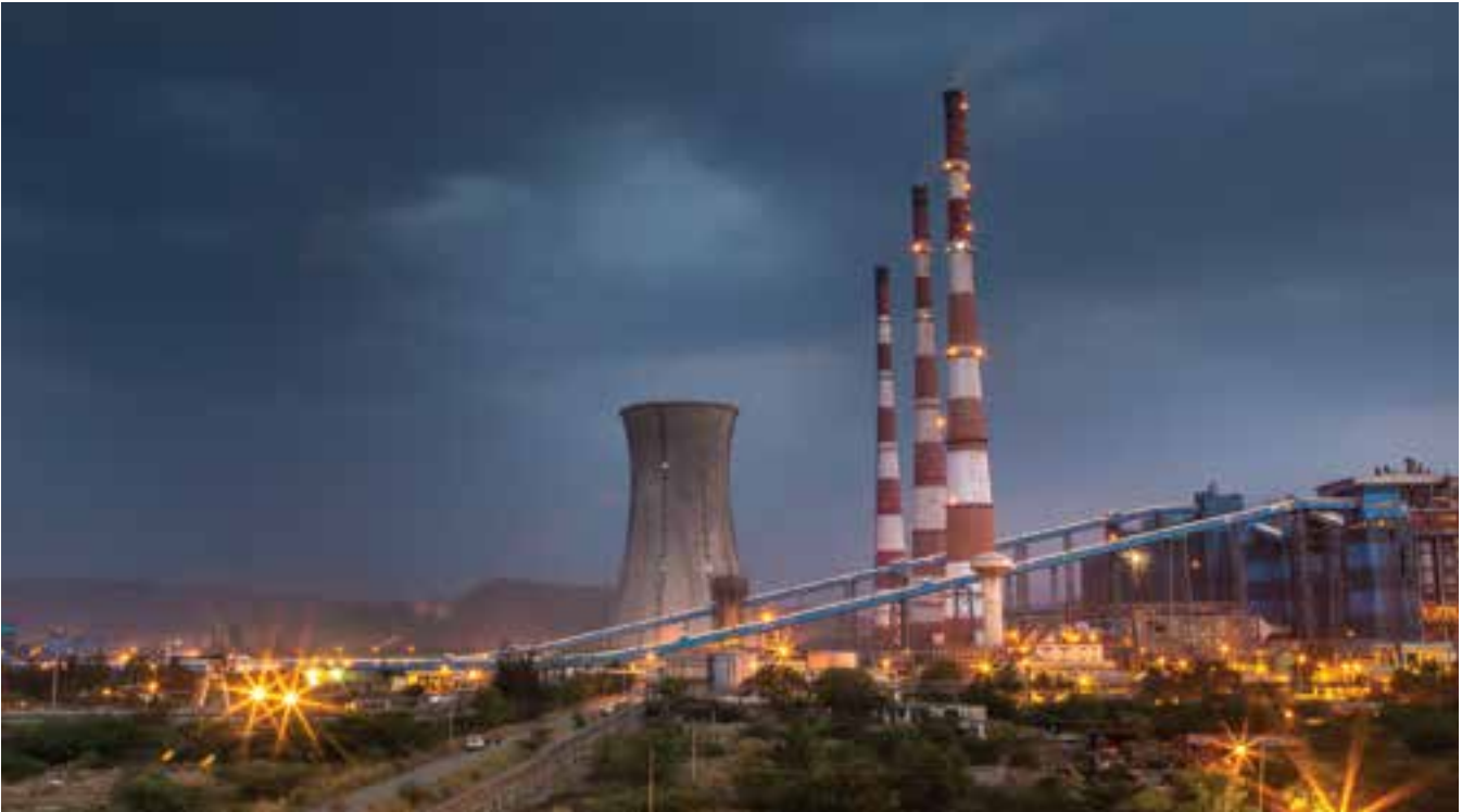
BHEL's first 700 MW supercritical thermal set commissioned at KPCL Bellary
