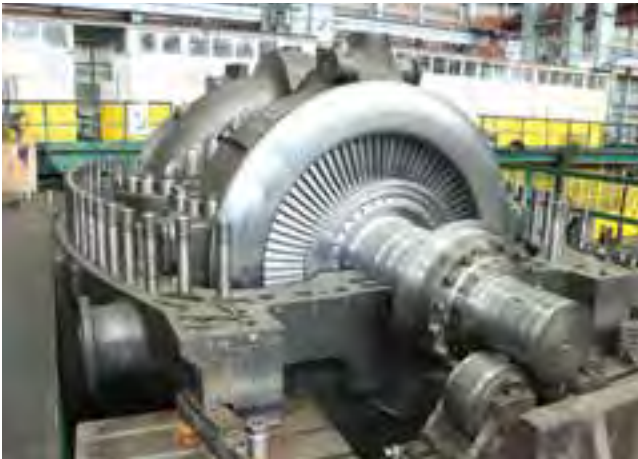
800 MW IP Turbine under assembly at BHEL works for NTPC Gadawara unit-2
